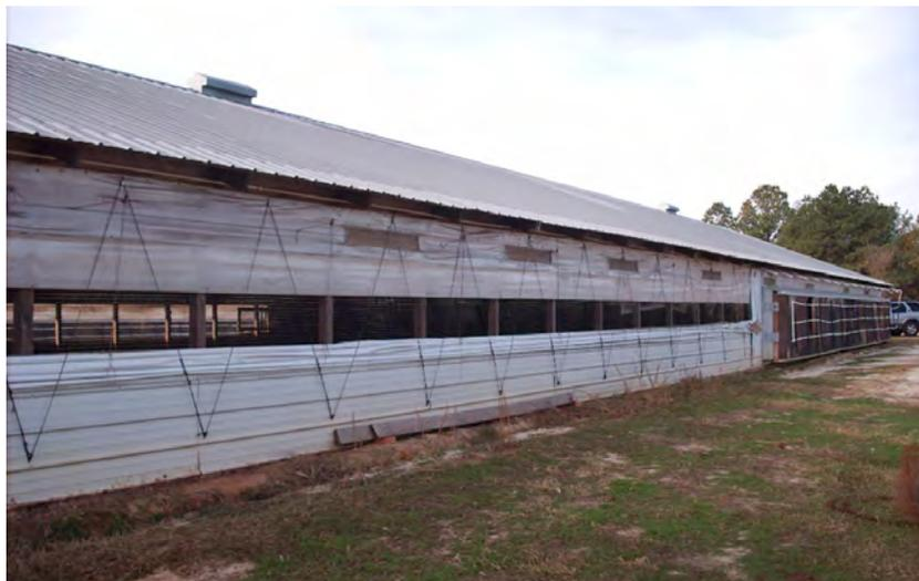
*Curtains can be lowered to provide natural ventilation.* Photo: NCAT
