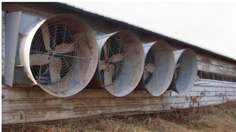
*Fans can help exhaust air and moisture out of a house.* Photo: NCAT
