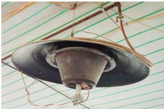
**Propane heaters can be suspended from the ceiling of a poultry house. Photo: NCAT**
