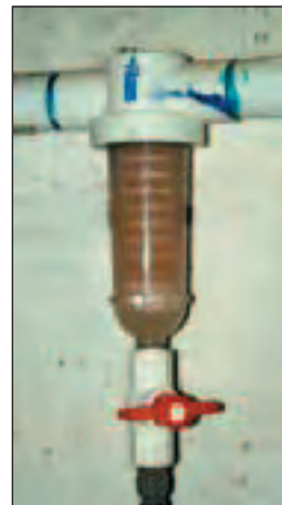
A Rusco strainer prevents crud from reaching the waterers. The flush-out valve at the bottom ejects the accumulated sediment without disassembling the strainer.
