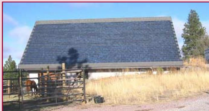
at sites that are far from the power grid. When the cost of roofing and the cost of power generation are both weighed in the balance, *building-integrated photovoltaics* (BIPV) can come out the winner for some locations (10).
