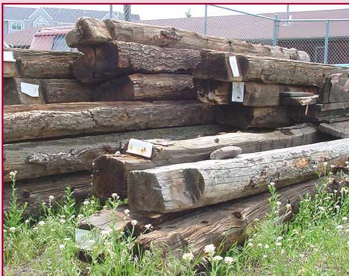
ing antique beams intact for reuse. If a farm building project involves demolition of an existing structure, it may be worth checking with a professional building-salvage operation to see whether there is market value for the materials.
