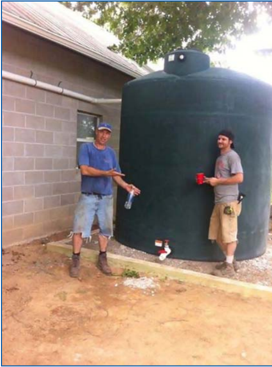
Newly installed cistern attached to farm building. Photo: Guy K. Ames, NCAT
