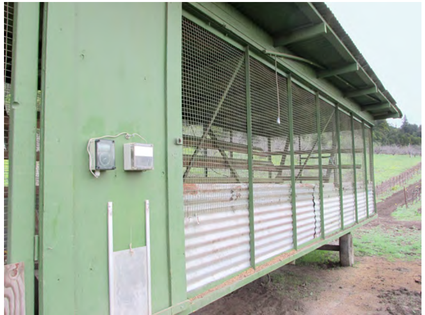
Housing that is well built will help to ensure the flock's safety. Installing automatic doors ensures reliable closing at night. Photo: Kevin Ellis, NCAT
