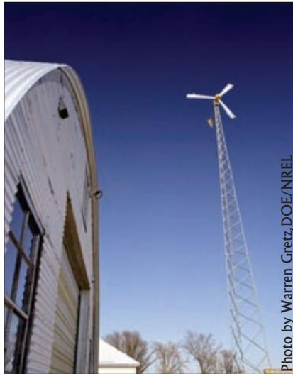
Small wind turbines, like this grid-connected Bergey 10kW Excel, can provide supplemental power for farms and ranches.
