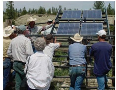
On the Ballard Ranch, the system's photovoltaic panels track the sun's movement for maximum solar exposure.
