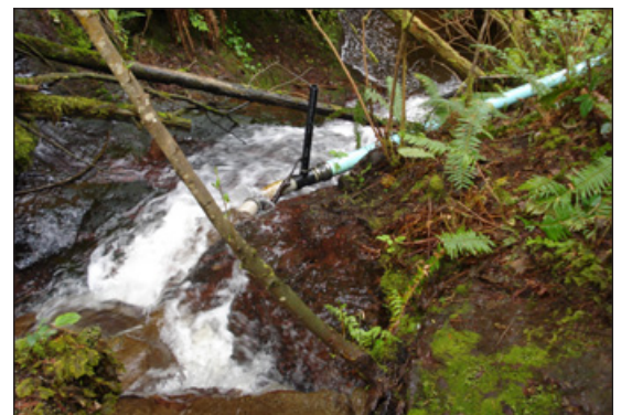
A micro-hydro intake and penstock temporarily divert a portion of the water flow and carry it to the location of the turbine. Photo: Leif Kindberg, NCAT
