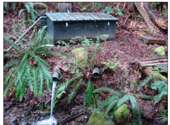
A “run-of-river” system returns flow to the same stream, reduces environmental impact, and generally eases the permitting process. Photo: Leif Kindberg, NCAT
