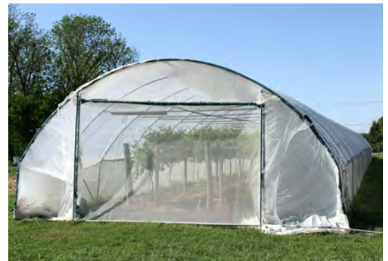
Research at the Arkansas Agriculture Experiment Station utilizes a 25-foot by 200-foot Haygrove Super Solo High Tunnel. Photo: Luke Freeman, NCAT
