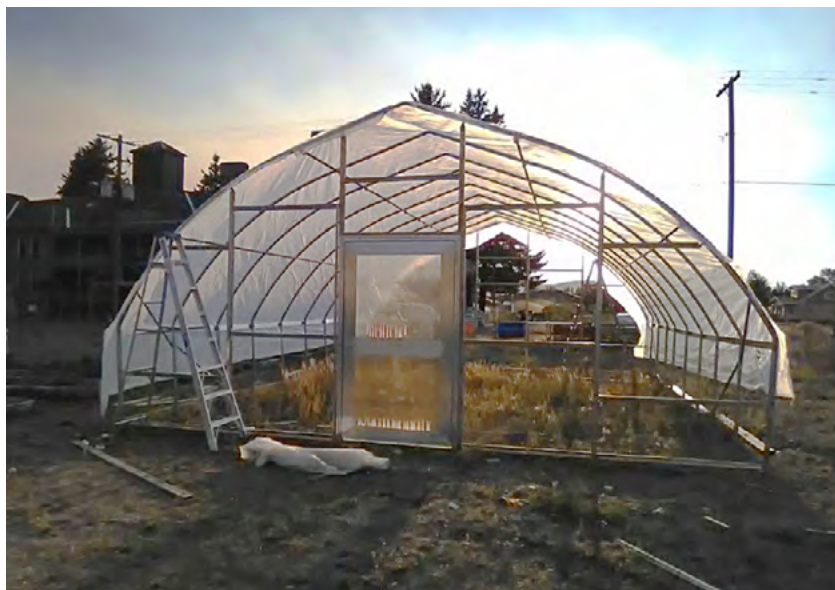
YMCA high tunnel close to completion. Photo: NCAT
