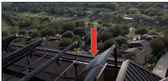
Solar collectors installed too close together, causing winter shading. Photo: Thomas Isaac, courtesy of Techsun Solar, Inc.
