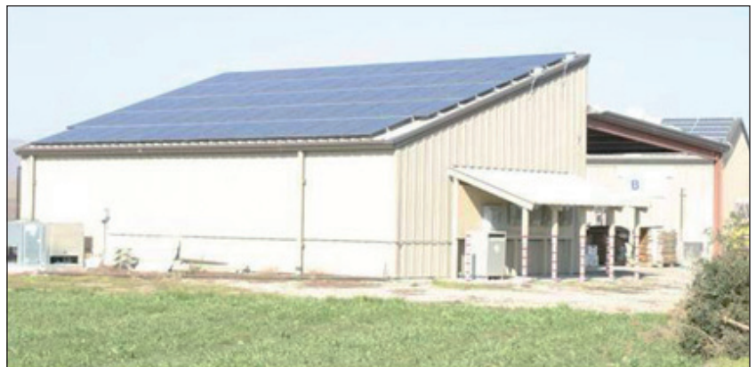
Solar arrays generating 10.8 kilowatts and 12.6 kilowatts greet visitors to this California organic vegetable farm. The arrays meet 25% of the farm's electrical energy needs. Photo: Mike Morris, NCAT
