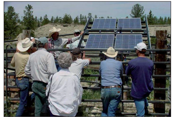
This 320-watt PV system in Montana pumps 5.5 gallons per minute from a 65-foot deep well, delivering enough water to meet the needs of 100 cow-calf pairs. The cost of its solar components was $5,500. Photo: Mike Morris, NCAT
