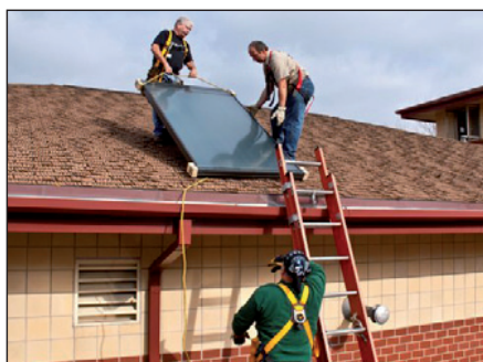
Installing a flat plate solar water heating collector. Photo: Courtesy of National Renewable Energy Laboratory
