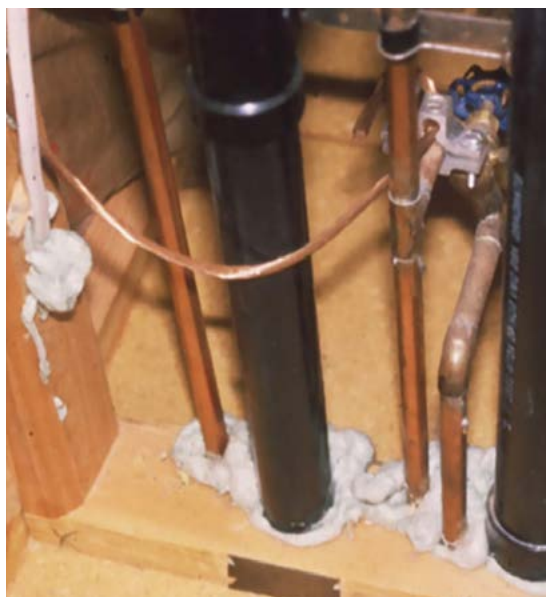
Figure 6. Well-sealed air leaks around plumbing. Photo: NCAT
