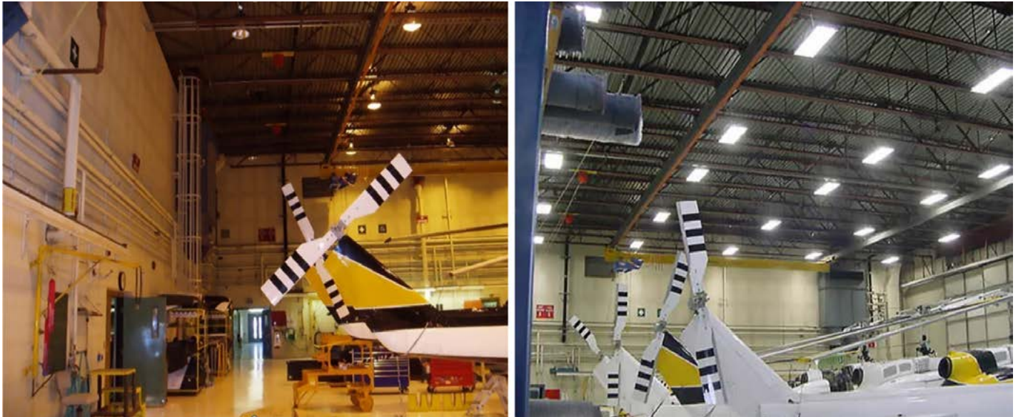
Figure 9. Lighting retrofit to LEDs with improved color rendering, efficacy, and efficiency. Photos: NCAT
